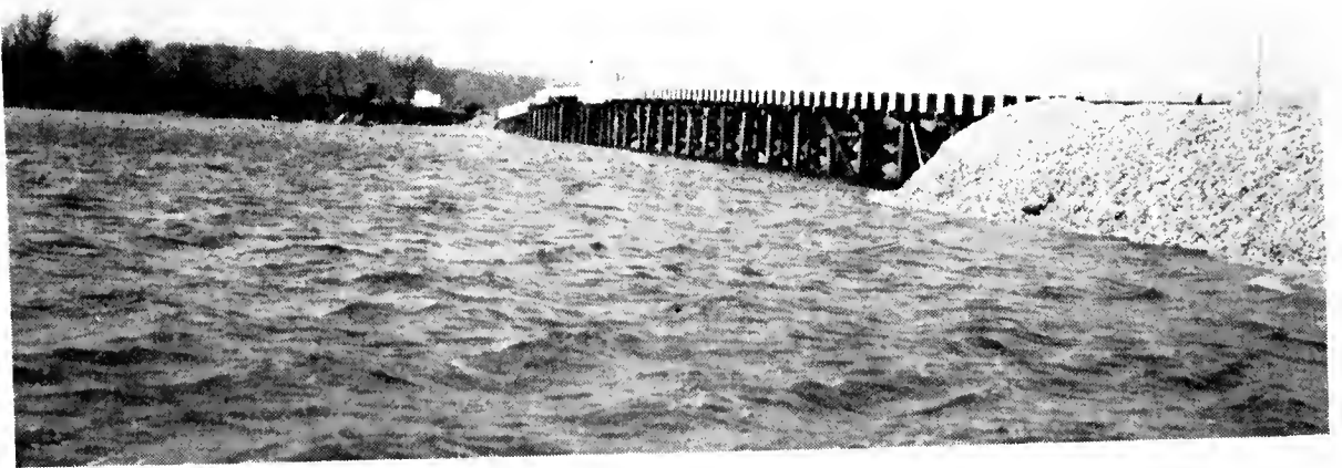
NEW WYE ISLAND BRIDGE
